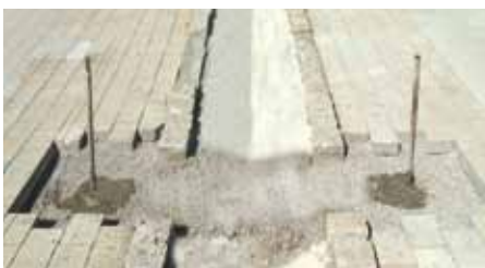
Completely installed injection piles
