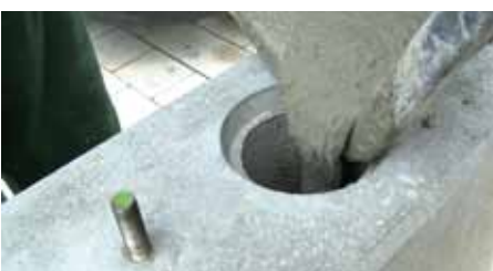
Grouting of the foundations
