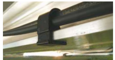
Cable guidance respectively cable duct
