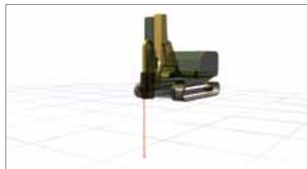
1. Drilling of the hole using a drill bit
